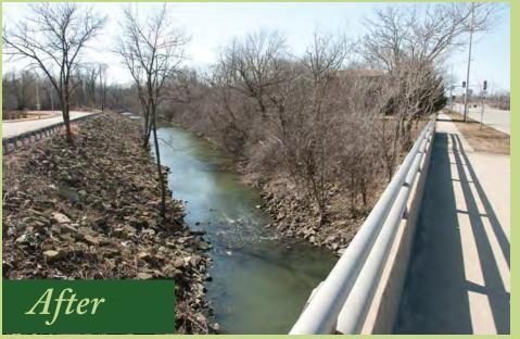
SSMP crews began clearing in February and were finished by March. After the area was cleared, it was seeded with native slope stabilization grasses before being sprayed with hydro mulch, a wet mixture of organic materials, to ensure proper growing conditions.
